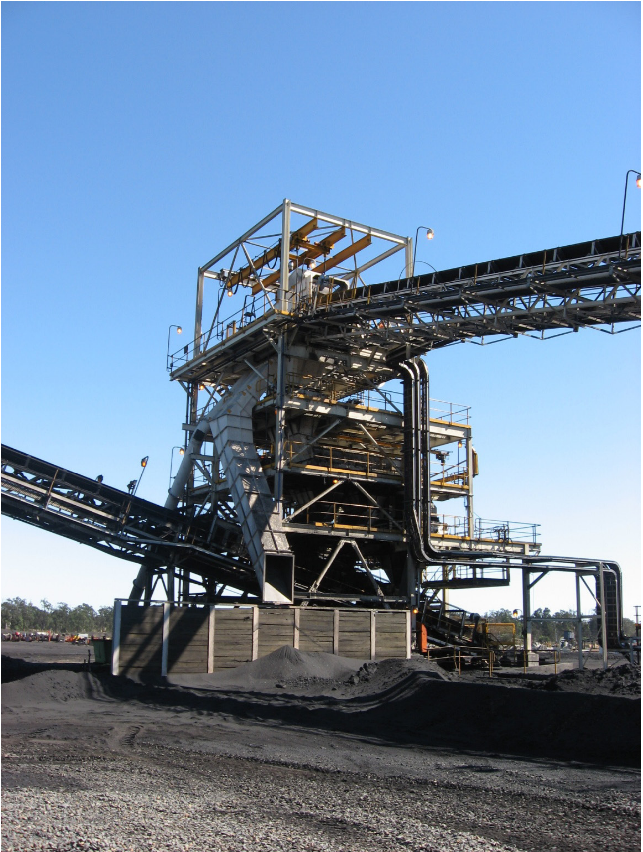
Plate 5. Typical Crusher / Sizer
